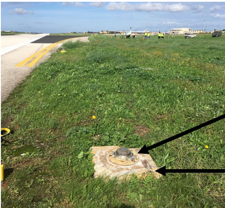
Fig. 7. Cause of punctured nose wheel tyre following runway excursion.
