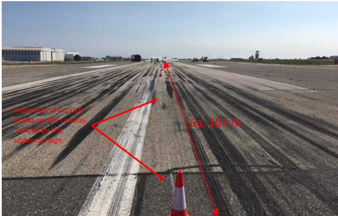
Fig.4. Superficial scratch marks on the runway as a result of the landing incident could be traced back to the final position of the aircraft.
