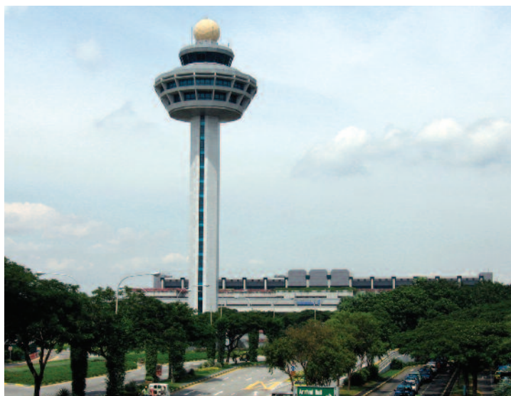
Singapore Changi airport, control tower
