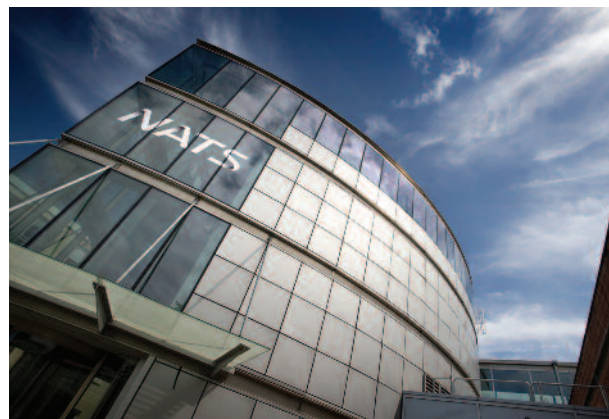
NATS UK Air Traffic Control, Prestwick Centre
