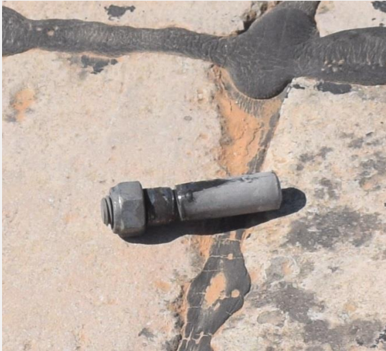
Figure 7: Close-up view of the remaining part of the retaining bolt found on RWY 23.
